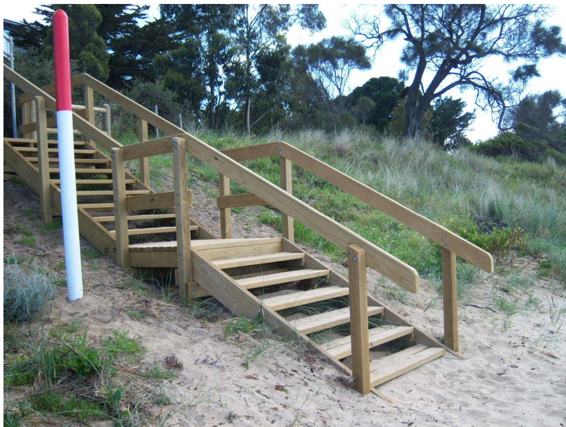
Figure 5: Example of an above-dune staircase installed at the Bellerive-Howrah Coastal Reserve.
