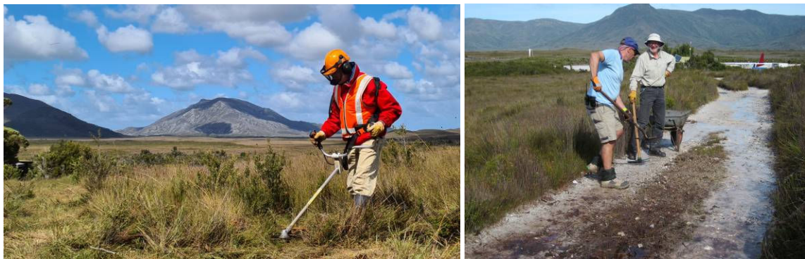
Routine maintenance jobs. Photos: Glenn Butterworth and Janet Fenton
