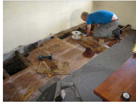
Head down, tail up. Willsons' west wing floor remediation. Photo: Chris Creese
