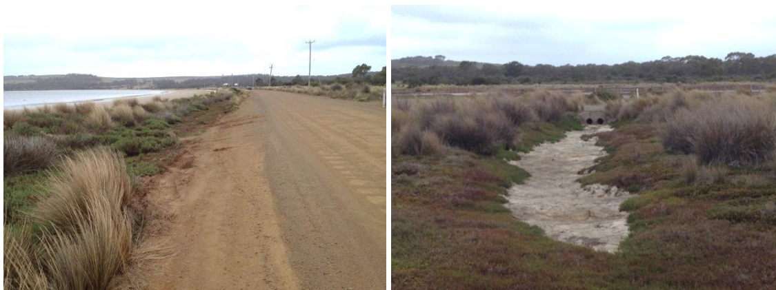
Figure 2. Left: Bicheno Street built over saltmarsh acts as an impediment for tidal flow separating the southern end of the Clifton Saltmarshes from Pipe Clay Lagoon. Right: The small drains under Bicheno Street have limited capacity in facilitating tidal exchange.
