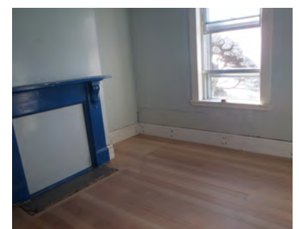
Replacement flooring in Quarters 2
