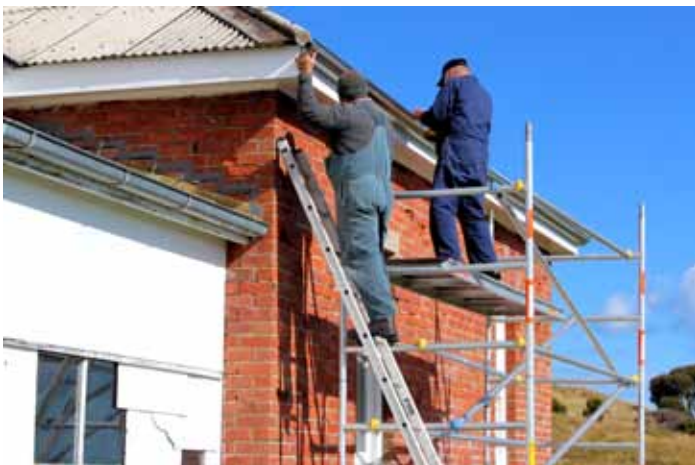
Keith Darke & Ron Fehlberg installing new gutters at Q1
