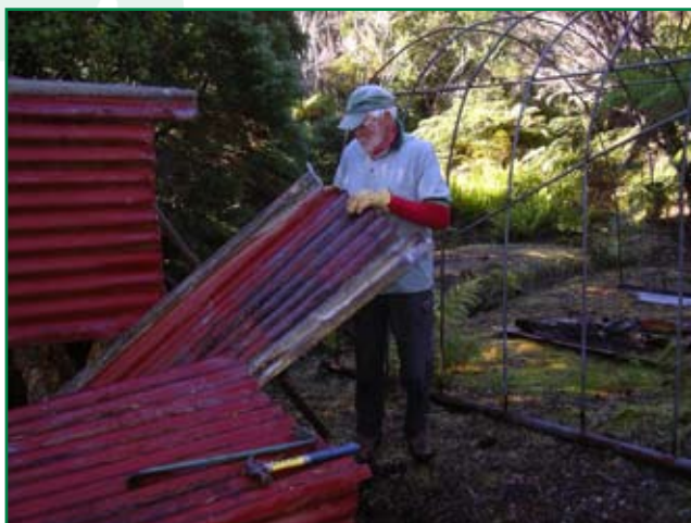
Repairs to the lean-to, Karina's (Janet Fenton).
