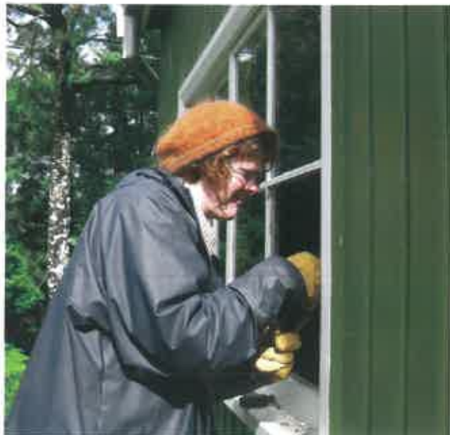
Qug removing broken glass at Claytons.
