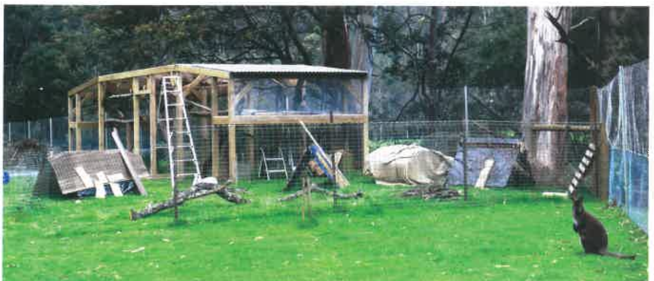
The works in progress are being observed by a local wallaby.
