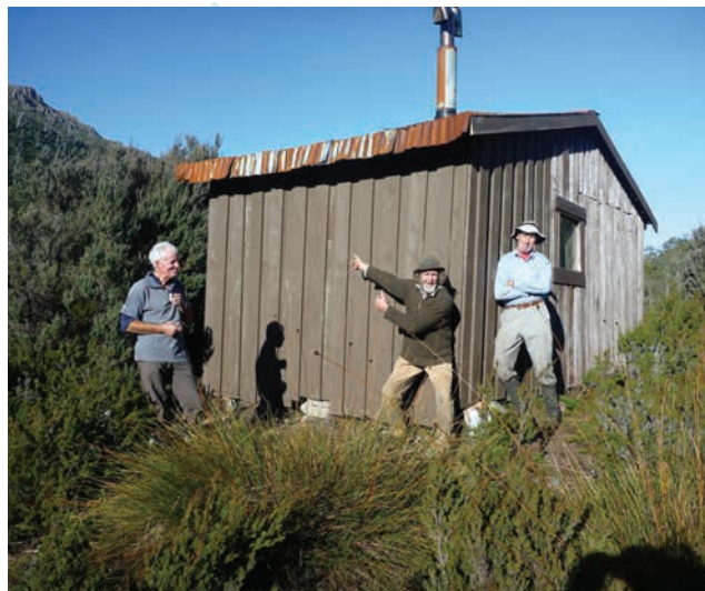
After the wall has been replaced – photo by Greg Kidd
