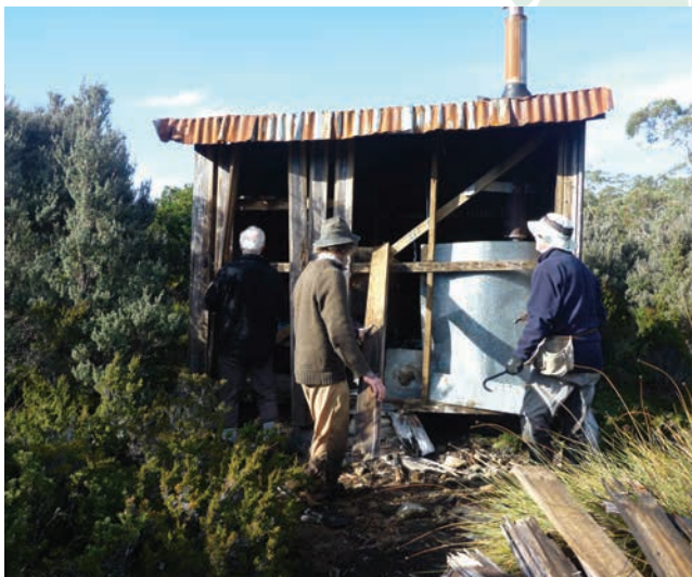
After removing the wall – photo by Greg Kidd
