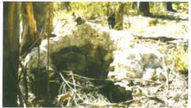
View of chimney showing stone base interior and clay capping (photo taken 2000) Photo Copyright K. Duncombe, FOBQS
