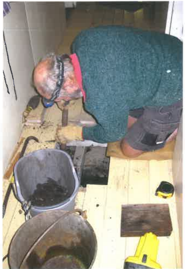
Jim at work on the King Fenton floor.
