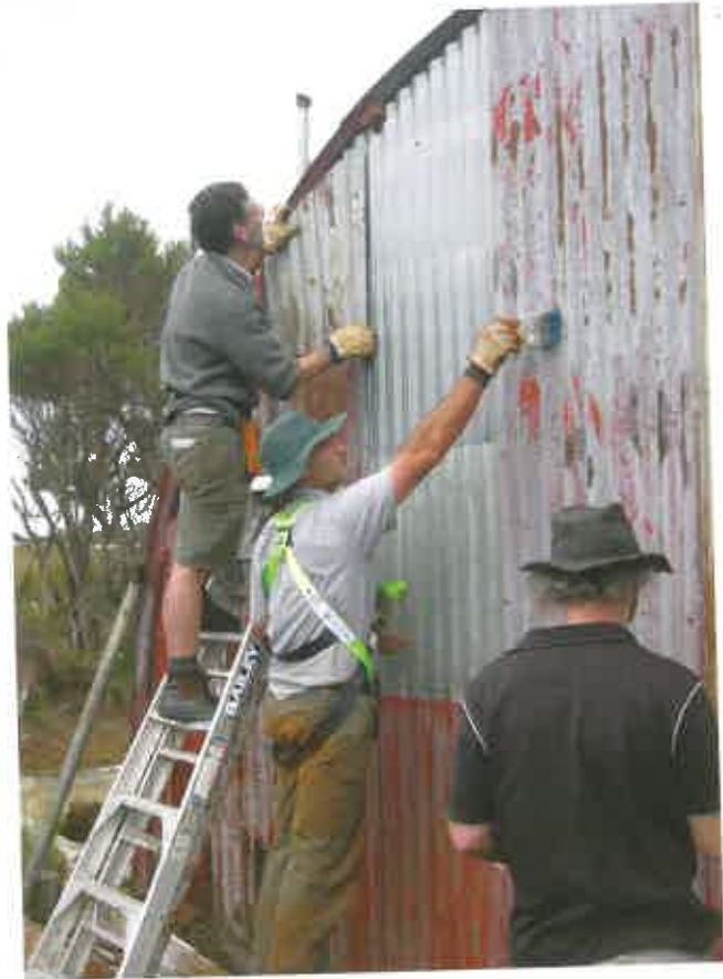
Red Shed back wall reconstruction with Ian, Jeremy and John.
