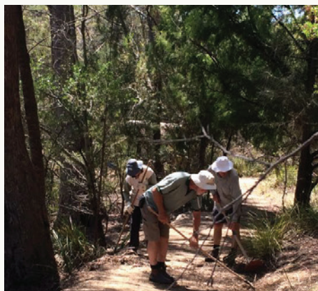
Clearing the track
