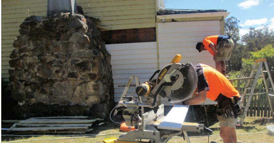
Replacing the timber on the homestead
