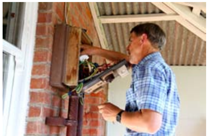
Andrew Boon Electrical work Q3
