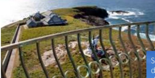
The wall at the left protected the keepers from the ocean swell
