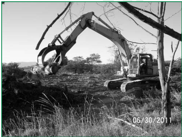
During – Logging in Progress
