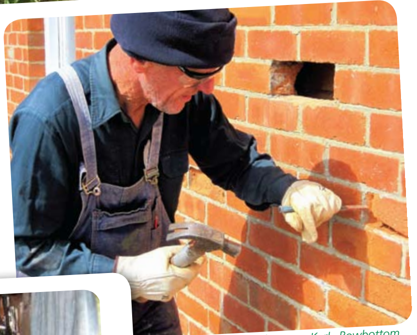
Former Tasman light keeper, Karl Rowbottom, working on eroded brickwork at Quarters 3. See story page 4.
