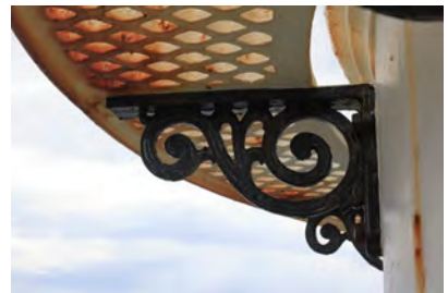
Funding secured for documenting work required for the light tower
