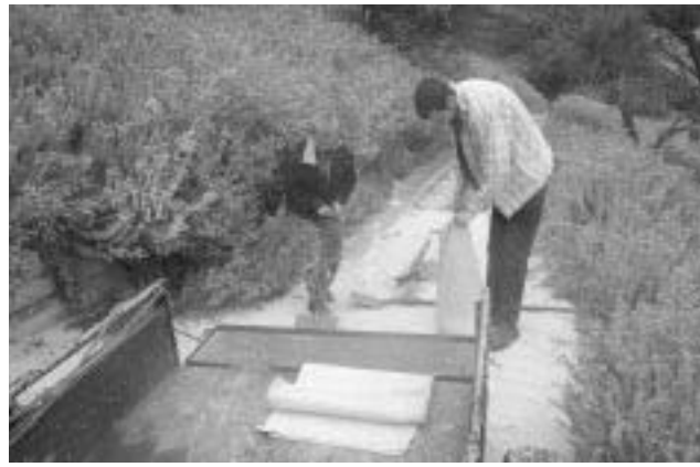
Filling sand bags for erosion control. Photo S Cronin.
