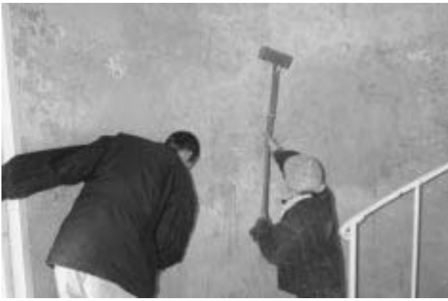
Cleaning lighthouse walls. Photo S Cronin.
