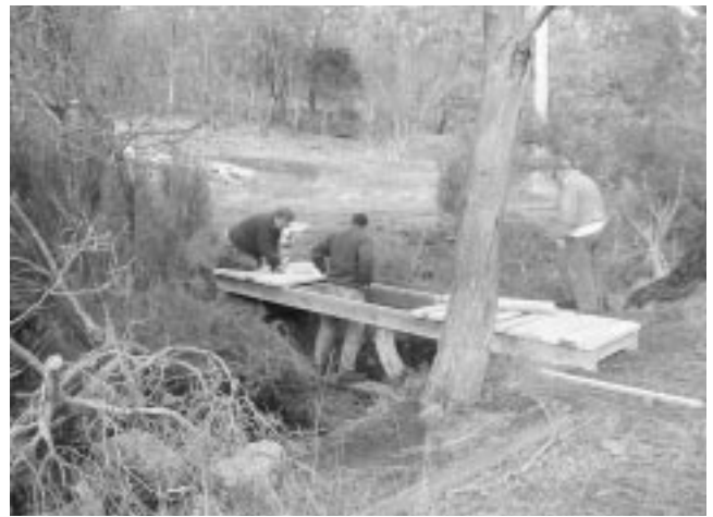
Constructing the bridge across the rivulet.
