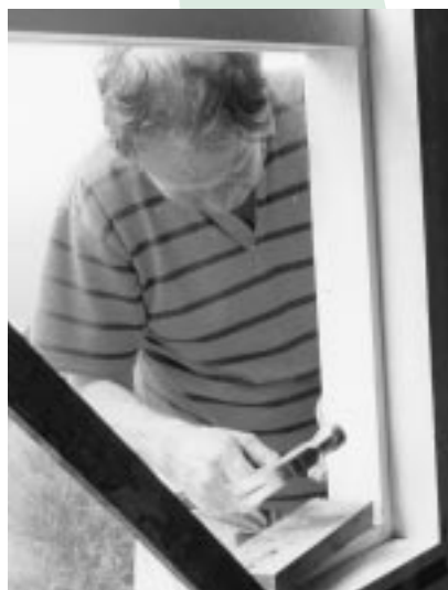
Alan Sanderson replaces broken window in generator shed. Photo C Bell.
