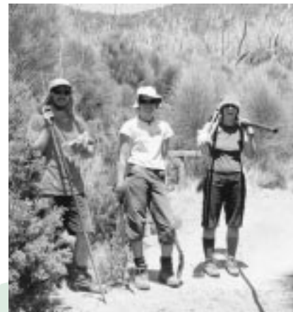
Paul Clark, Sarah Lovibond & Esther Staal undertake repairs to lighthouse track on Deal Island. Photo C Bell.
