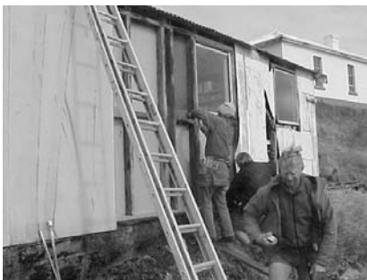
Maatsuyker volunteers replacing cladding on workshop wall.
