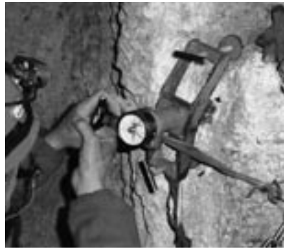
Testing a Newly Installed Bolt at Midnight Hole
