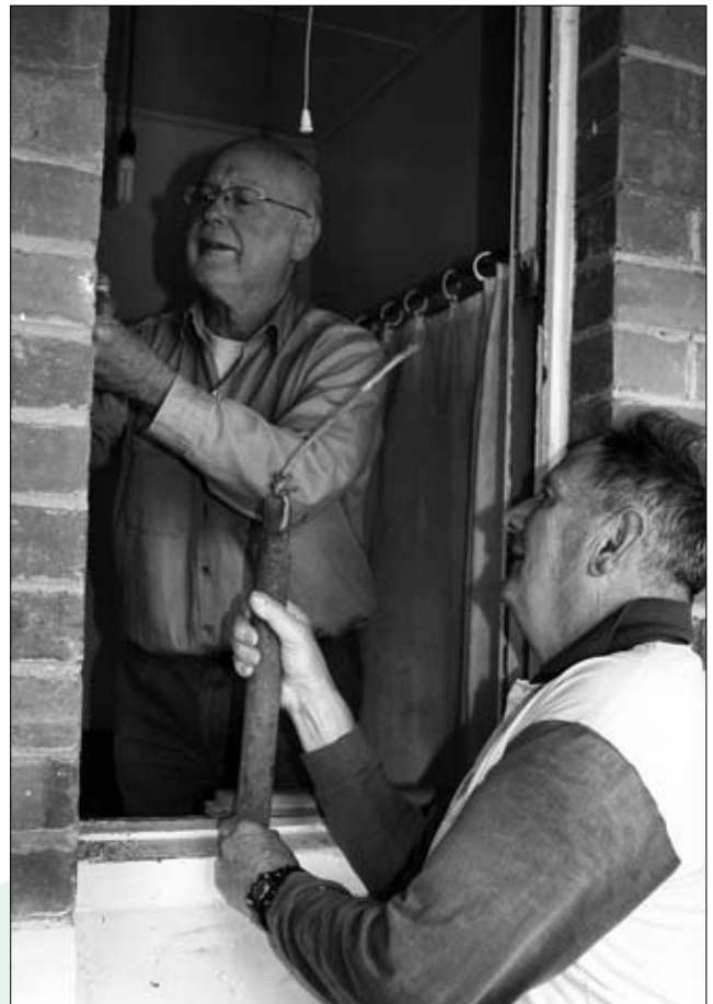
Kevin Heaton and Alan Sanderson Repairing Window in Q3 Tasman Island
