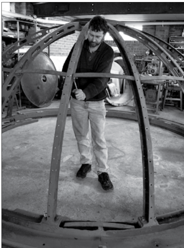
Chris Creese Reassembling Domed Roof of Tasman Island Lantern Room in Hobart
