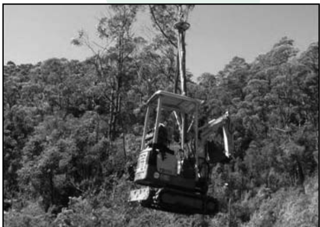
Excavator Arrives at Frenchmans Cap
