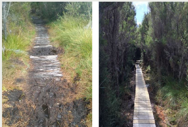
FRENCHMAN'S CAP BOARDWALK IMPROVEMENTS
