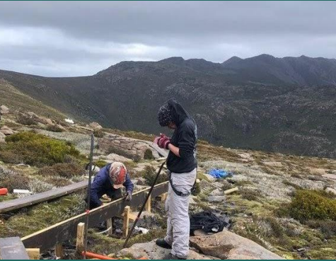
Installing planks Photo from John Hughes
