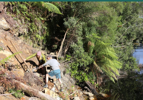
Friends of the Franklin Landslip repair
