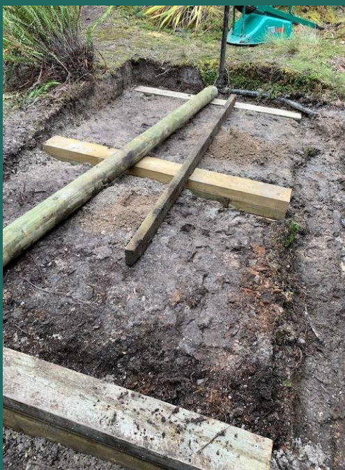
Prep for the new tank-stand
