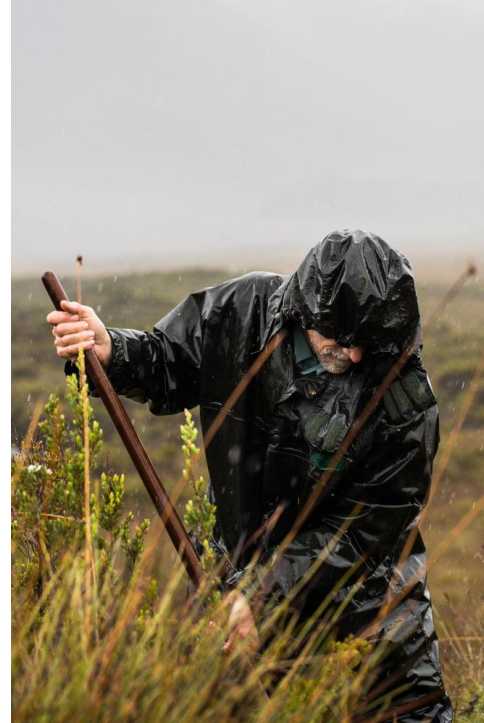
There's not stopping David on the drains
