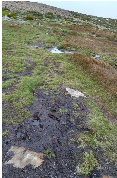
Site before planking showing damage
