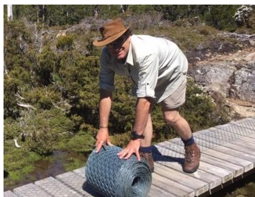
Laying wire on Rodway Track Boardwalk
