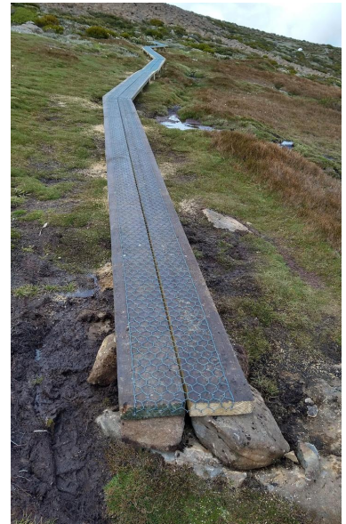
Site after timber added
