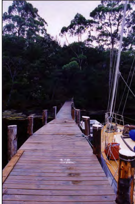
Illustration 1: View along the jetty constructed in 1998. (Photo: D. Parham March 2002).
