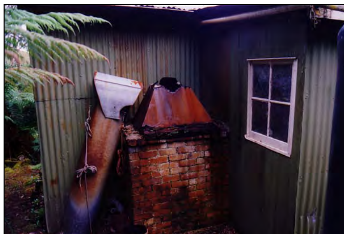
Illustration 12: View of the original external chimney showing the flue assembly which was part of the intake at the Ray River mines until it was salvaged and adapted for domestic use by Clyde Clayton.
