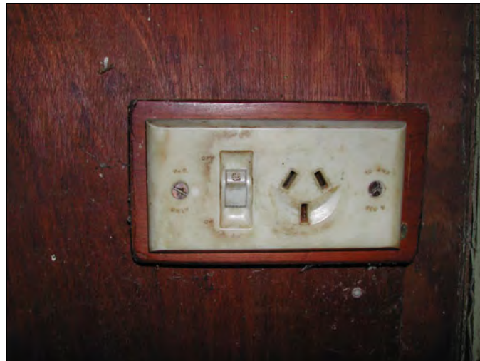
Illustration 19: Original powerpoint detail. (Photo: D. Parham, February 2003).
