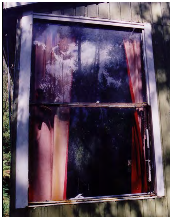
Illustration 5: Window to lounge in north end wall (this is W2 in Appendix 4). Note: The entire north wall has been replaced and a new window to match the original (pictured above) is being fabricated. (Photo: D. Parham, March 2002).
