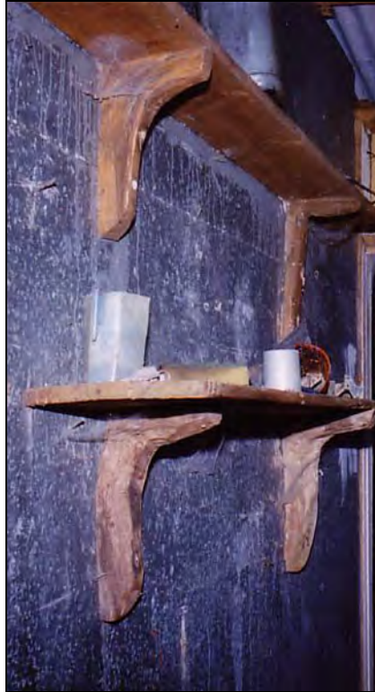
Illustration 22: Laundry shelves supported on tree 'knee' brackets made by Clyde Clayton. (Photo: D. Parham, March 2002).
