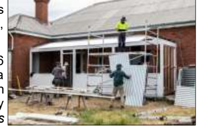
Construction at Q2 underway ...
