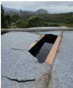
Repairing wind damage to tank at Q3
