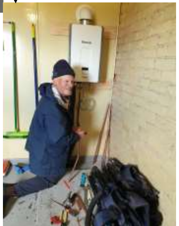
↓ Ron installs the new hot-water heater
