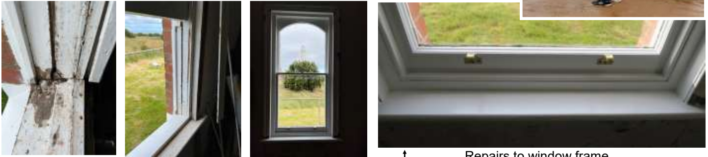
Repairs to window frame. Note the polished sash pulls !
